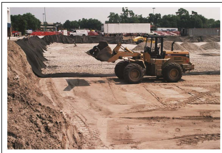
Figure 6 Installing foundation layer
