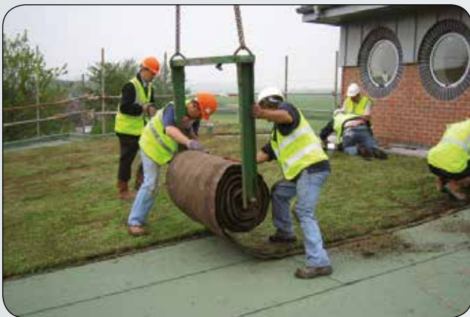
Long length rolls being craned into position and installed.
